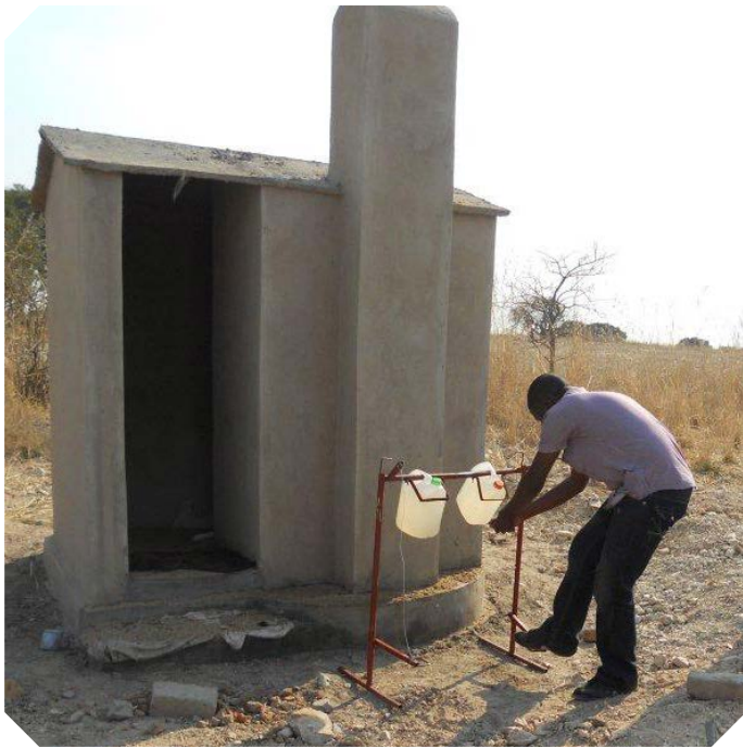
Ventilated improved pit latrine and handwashing station
